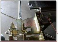
Clamp door bracket to the front lip level with the edge of the door. Drill 13/32" holes in center of each slot.
