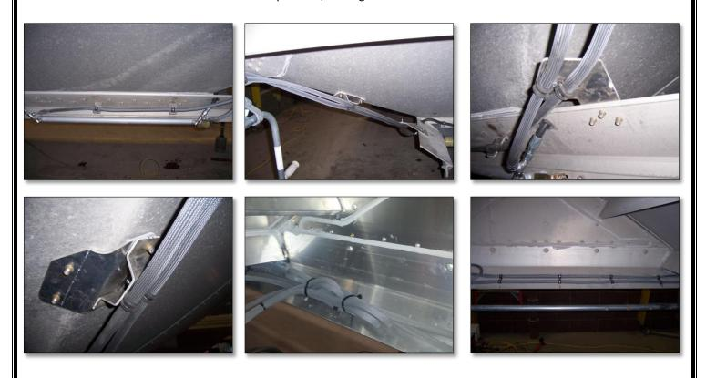
vii. After all hoses are mounted and secured, tighten all fittings.
