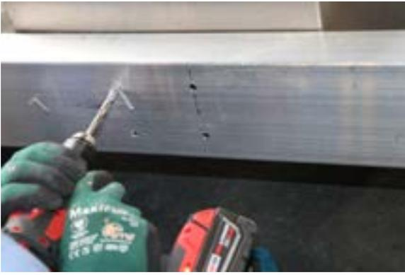
Place the .386 drill bit into the power drill and drill out the four marked holes.
