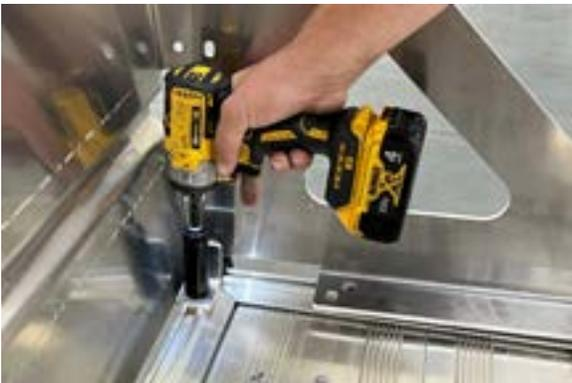
Place 4 angle supports on the front side of the trailer (2 on bottom and 2 on top). Connect your angle supports to the side posts by inserting four 2 3/4" bolts through the side posts and fasten loosely using 11/16" wrench. Fasten the two angle supports on the bottom to the L-track studs using 1/2" wrench.
