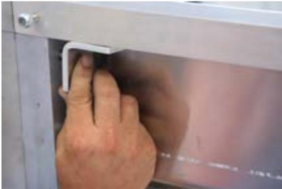
Attach front cross member to the top angle supports by inserting two 2 1/2" bolts from the top side, and fasten loosely using 11/16" wrench.
