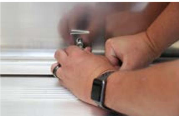
Add an additional L-track stud for new side panels. Discard L-track washer.
