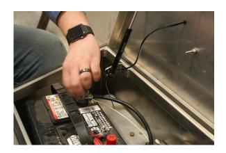
Using your crimping tool crimp the wire and place electrical connectors to wires. (Black wire from solar panel leads to negative terminal of battery, black/white wire leads to positive terminal of battery).
