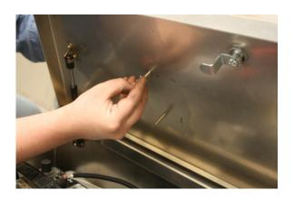
Slide your 3/4" bolts through from the top side of the toolbox, and place the washers and fasters onto the four bolts from the bottom side.
