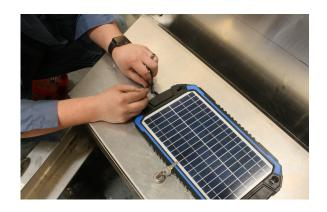
Next, place rubber grommet into the drilled out hole so that no water is able to enter the toolbox.
