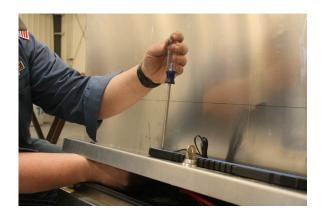
Tighten bolts using your 3/4" wrench and screwdriver until all four bolts are tightly fastened.
