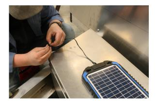
Place rubber grommet over the cut end of the wire and thread it down to the drilled out hole.
