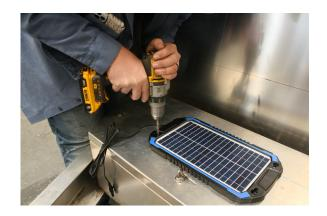
Next, 1" from the middle of the cord side of the solar panel drill a hole to thread cord through to the battery.
