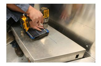
Place 5/16" drill bit into the power drill and drill out the four marked holes.
