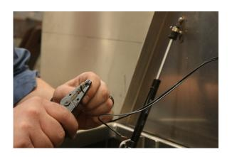
Using your wire cutters, cut the wire from your solar panel to your desired length so it reaches the battery.
