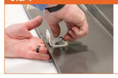
Attach (2) 1/8" AL L-Brackets to the bottom of the front panel with a 3/4" bolt. Slot is on the deck.
