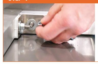
Use a 2 3/4" bolt for horizontal connection through the side panel, side post, front panel, and L-Bracket.
